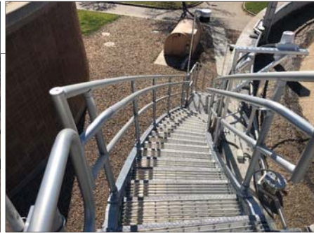
New staircase to new primary anaerobic digester #3.
