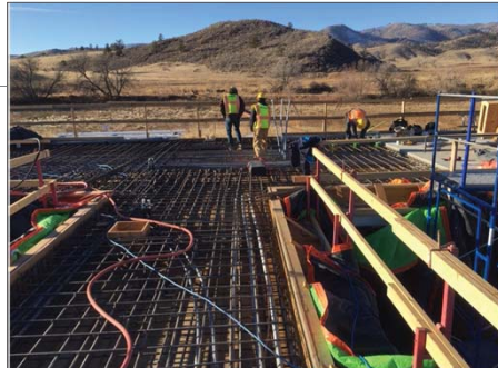
Rebar for Operating Floor
