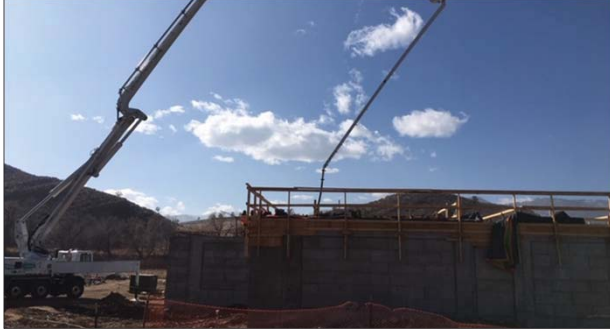
WTP Concrete Floor Being Poured
