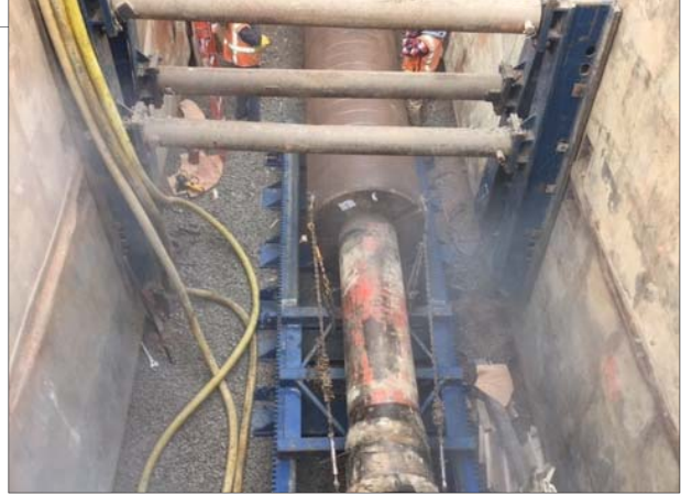
Boring Shaft UPRR Guided Pipe Hammer
