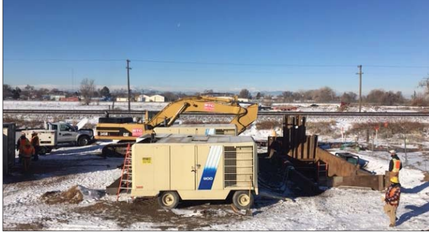
Boring Pit UPRR
